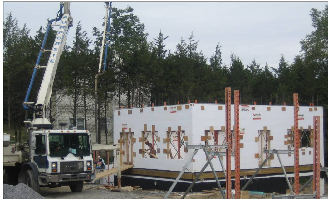
Concrete Poured into Stacked Insulated Concrete Forms
